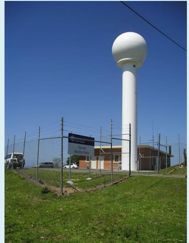
Modern weather RADAR unit
